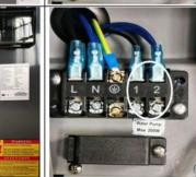
Water Pump Wiring:
