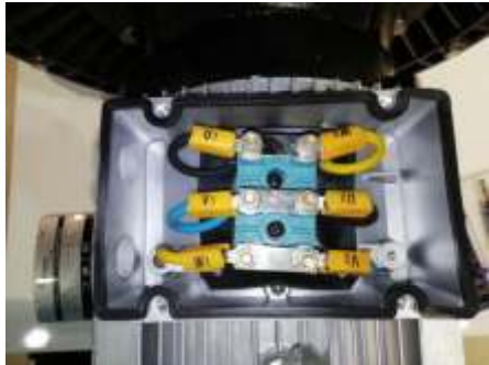
The factory connection is a Dealta connectiton
