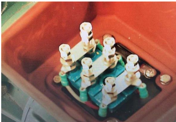
The factory connection is a Dealta connectiton
